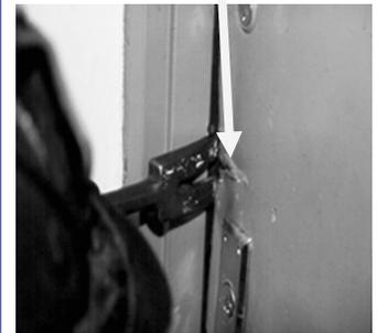
When forcing outward opening doors the bevel goes toward the frame.
